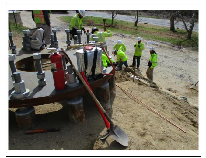
**Photo 3:** A set of fire tools (5-gallon backpack pump, round point shovel, Pulaski, and 2A10BC fire extinguisher) was observed at active construction sites in accordance with APM HAZ-01 and APM HAZ-04 during ground wire and rod trenching at Z118106 (TL 682).
