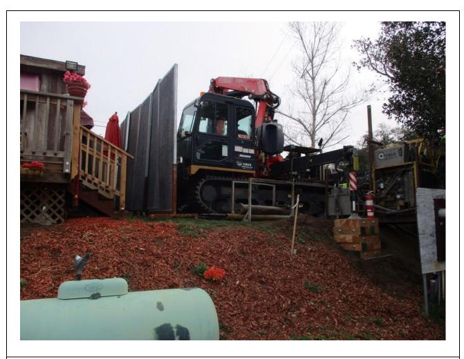
**Photo 5:** Noise barriers were observed being used during micropile drilling activities at Z118042 (TL 682) to minimize noise disturbance at an adjacent residence, in accordance with MM NOI-1.
