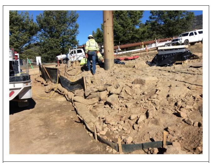
**Photo 4:** During capping at Pole Z118051 (TL 682), erosion control BMPs were observed to be in need of maintenance. The project Lead Environmental Inspector was notified, and BMPs were subsequently repaired.
